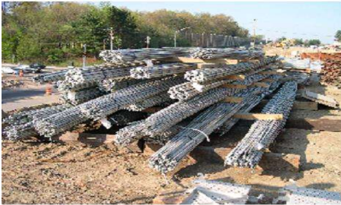
Stacking of Reinforcement at Construction site
